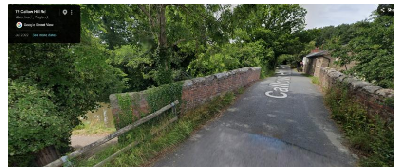
Image looking northwest along Callow Hill Road from the southern side of the bridge (site on the left)
