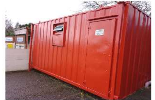
Figure 1: Existing 'portable' toilet block at football ground. Approx 3m x 5m Installed as second-hand unit approx 10 years ago. This unit comprises of a single female toilet one end and 3 cubicle male toilet plus 5 urinals at other end.
