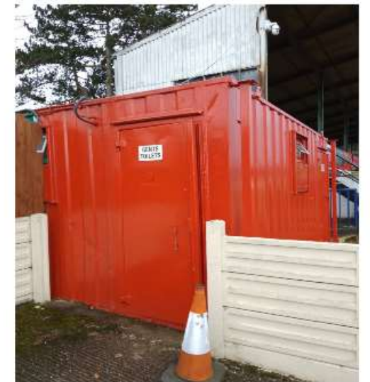
Figure 1: Existing 'portable' toilet block at football ground. Approx 3m x 5m Installed as second-hand unit approx 10 years ago. This unit comprises of a single female toilet one end and 3 cubicle male toilet plus 5 urinals at other end.
