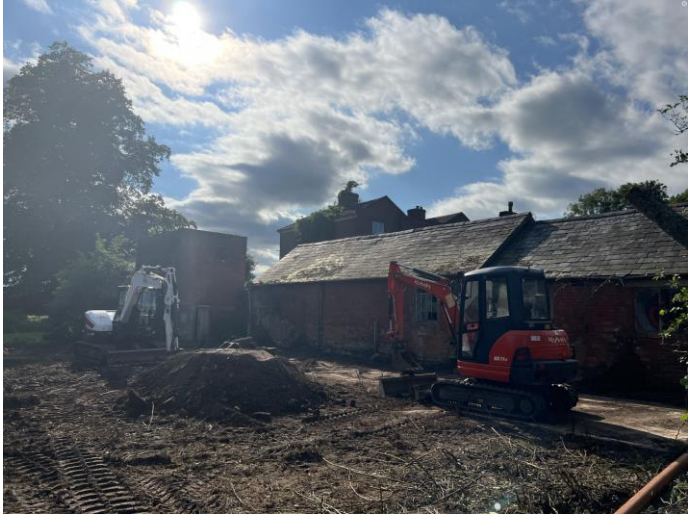
View towards unit 4 and drainage trenching
