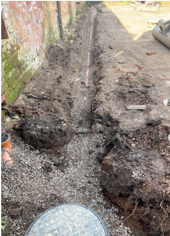
Drainage trenching to the rear of unit 4
