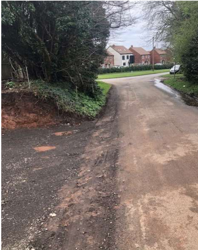
Travelling south along Blackwell Road (new access as constructed)
