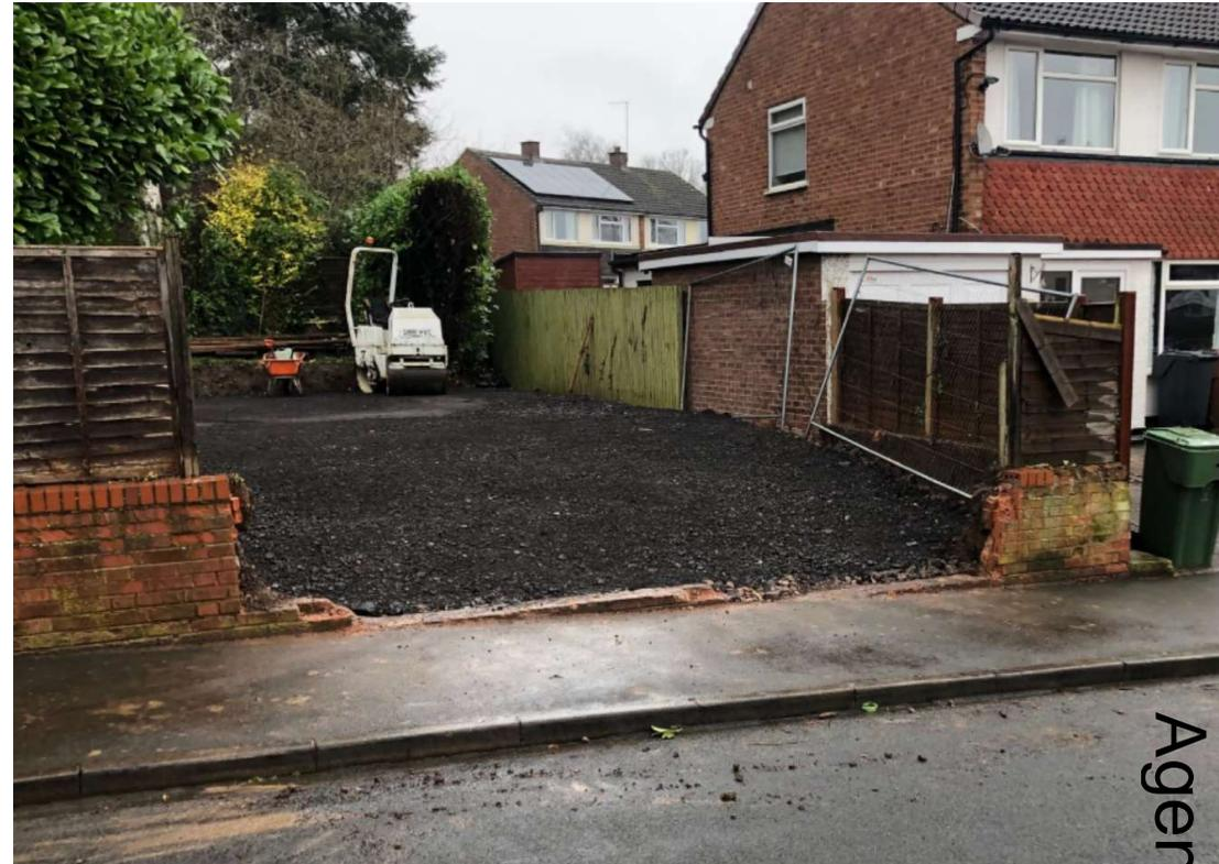
Photo of site following part removal of dwarf wall and fence
