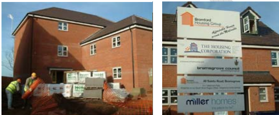
Eight Flats for Young People Completed May 2005
